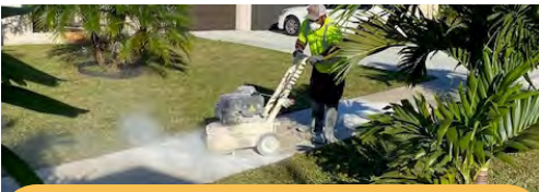
SIDEWALK & ASPHALT REPAIRS
