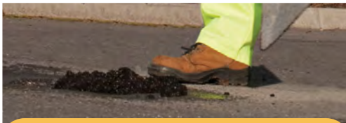
PAVEMENT MAINTENANCE & REPAIR
