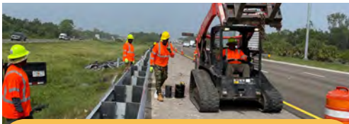
GUARDRAIL INSTALLATION, MAINTENANCE, & REPAIR
